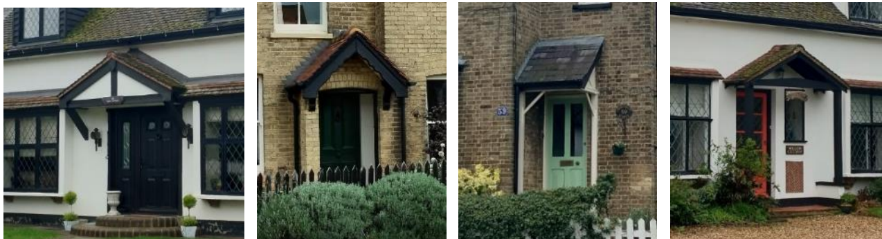
Fig. 5.23: Examples of existing canopies
