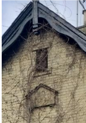
Fig. 5.18: Gable-end vent and stone plaque
