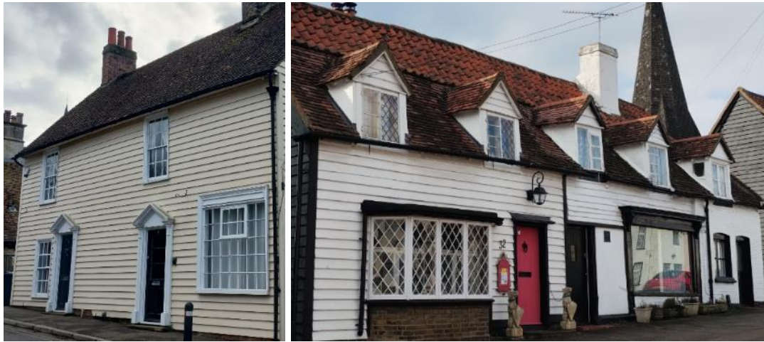
Fig. 5.8 & 5.9: Significant window alterations
