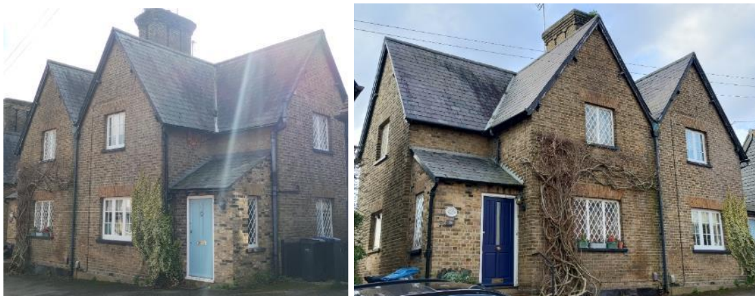
Fig. 5.22: Semi-detached house viewed from both sides
