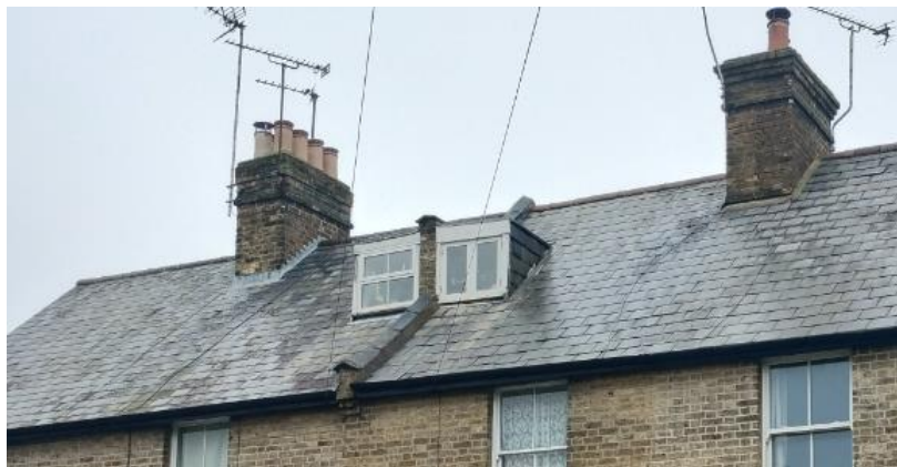
Fig. 5.2: Chimney and dormer window alterations
