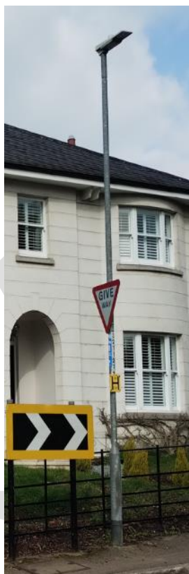
Fig. 8.1: Example of inappropriate street lighting
