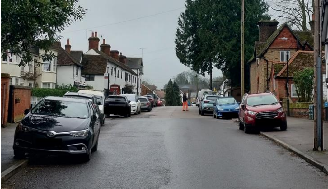
Fig. 5.3: Cars parked on the road, many partially on the pavement
